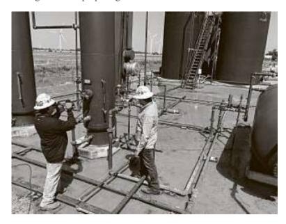
Courtesy OTA Environmental/ A Lead Detection and Repair crew surveys a production facility.
